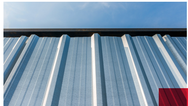
Figure 4: Structural metal roof panel system over insulation fitted between thermally broken framing, over steel or wood decking
