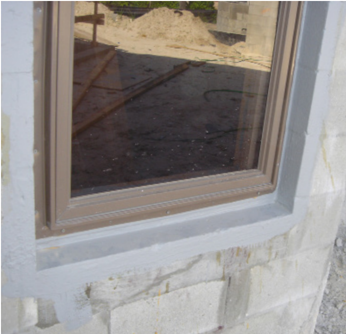
Photograph 2: Fluid Applied Flashing - You absolutely must use a fluid applied coating around the entire perimeter of the rough opening.
